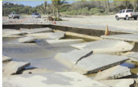
*Figure 2: Destruction to the Vieux Fort Highway caused by seawater inundation. Without action more intense storms brought on by climate change will continue to cause costly damage to infrastructure. (Source SLNT)*
